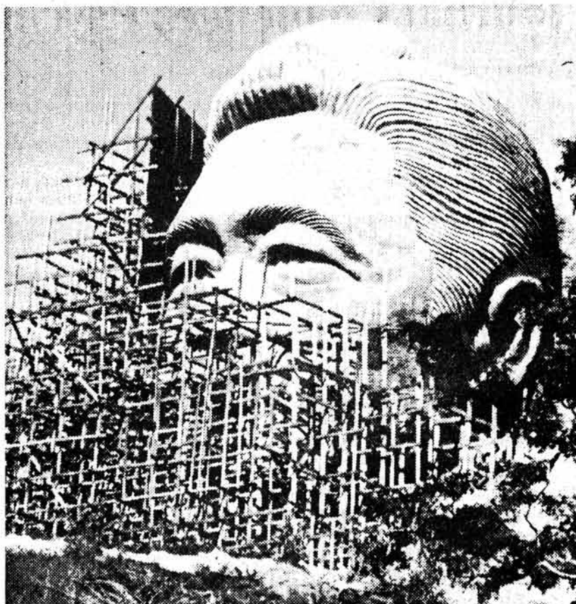
Statue of Ferdinand Marcos being built north of Manila.
