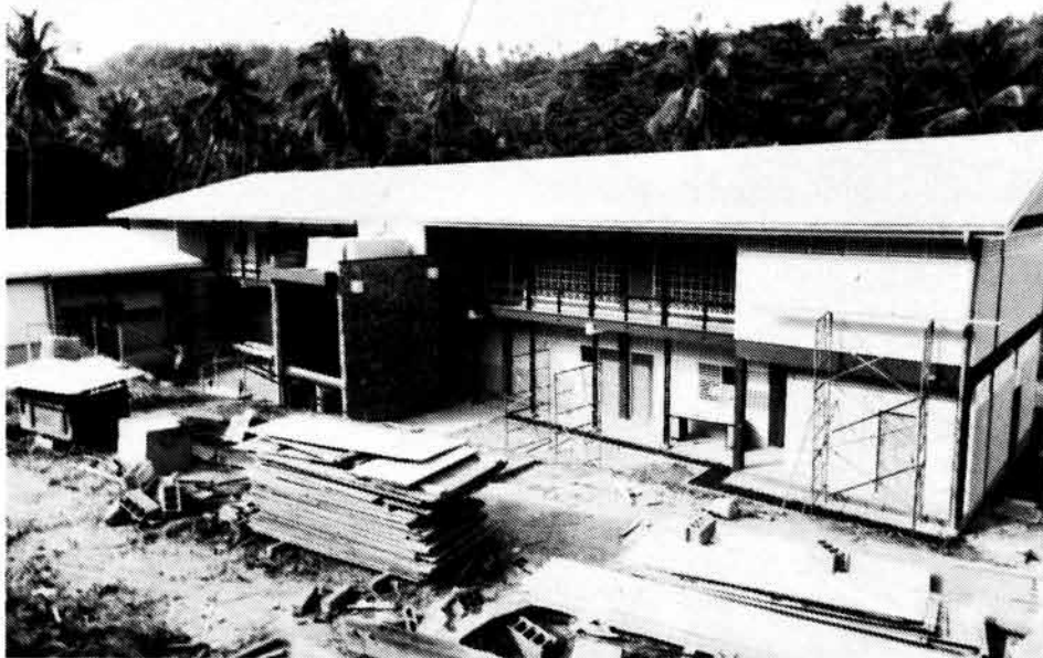
New elementary school under construction in St. David's.
