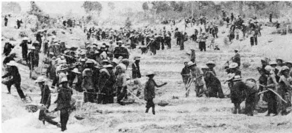
Work brigade constructing irrigation dikes.
