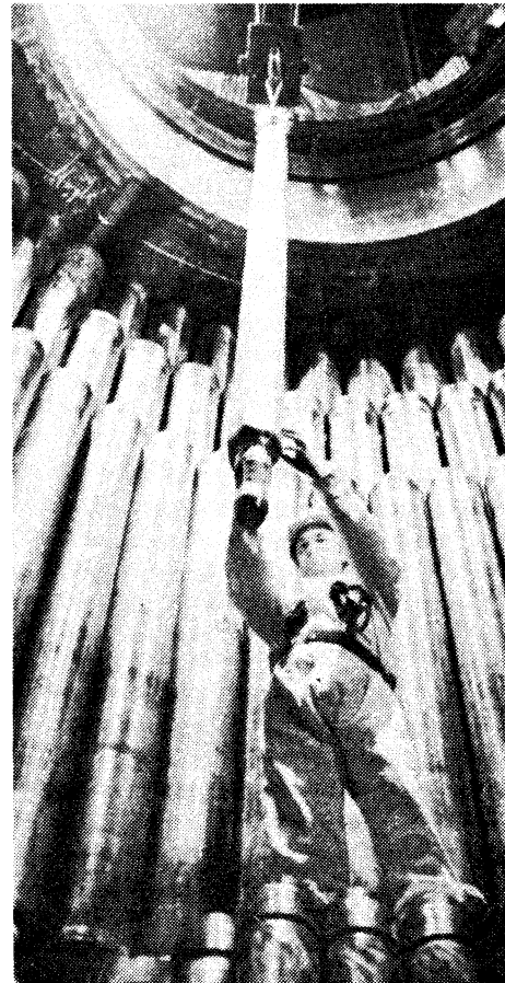
Inside the reactor. Once in operation, this core must be continually cooled or a meltdown will occur.
